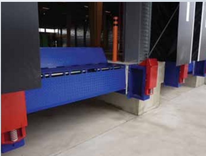
The truck is docked, the door is open but a pallet placed at the end of the trailer prevents full deployment of the leveler ...
