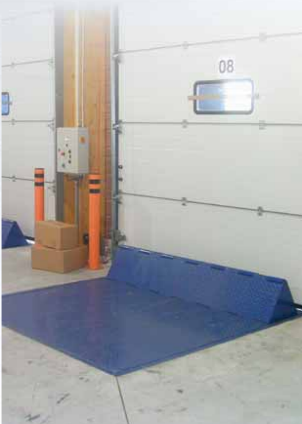
The refuge area, allows to protect a careless person from being crushed, here per example, the second driver who is knocking on the door of a warehouse while his colleague moves back to dock.
