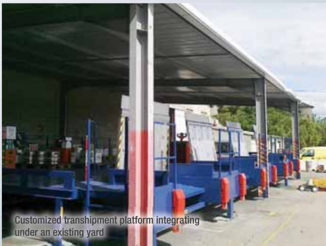
Platform with stationary yard ramp, equipped with aluminium drawbridge levelers type 8860 and a covered structure
