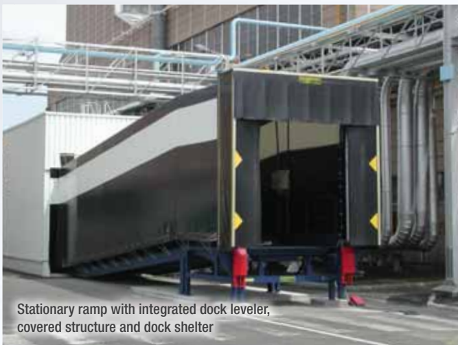
Stationary ramp with inlet structure and integrated dock leveler
